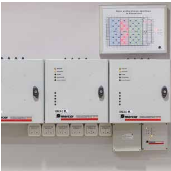
Fig. 2 Example of electric smoke exhaust control system
